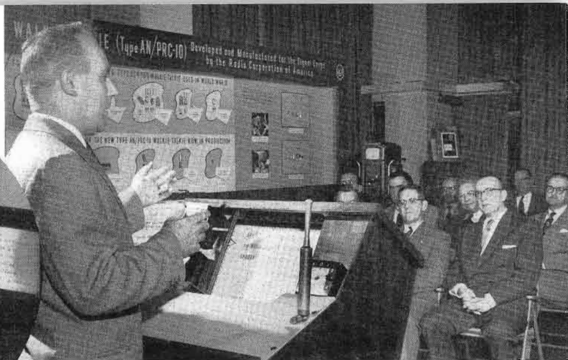
A Teleprompter user, reading his speech as it unrolls before him, is able to make his delivery sound extemporaneous. At left: An operator in the wings, working from an identical typewritten version of the text, adjusts the speed of the Teleprompter to the vocal speed of the speaker.
